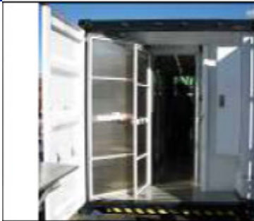
7 Racks plus Network
