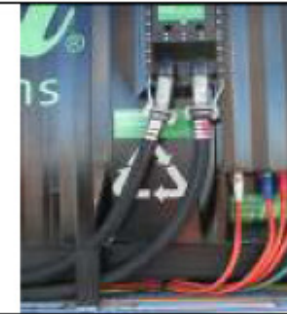
Data Power Cooling
